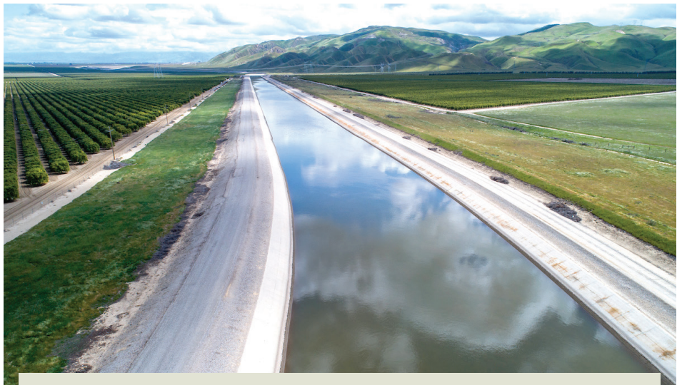
State Water Project California Aqueduct Credit: California Department of Water Resources
