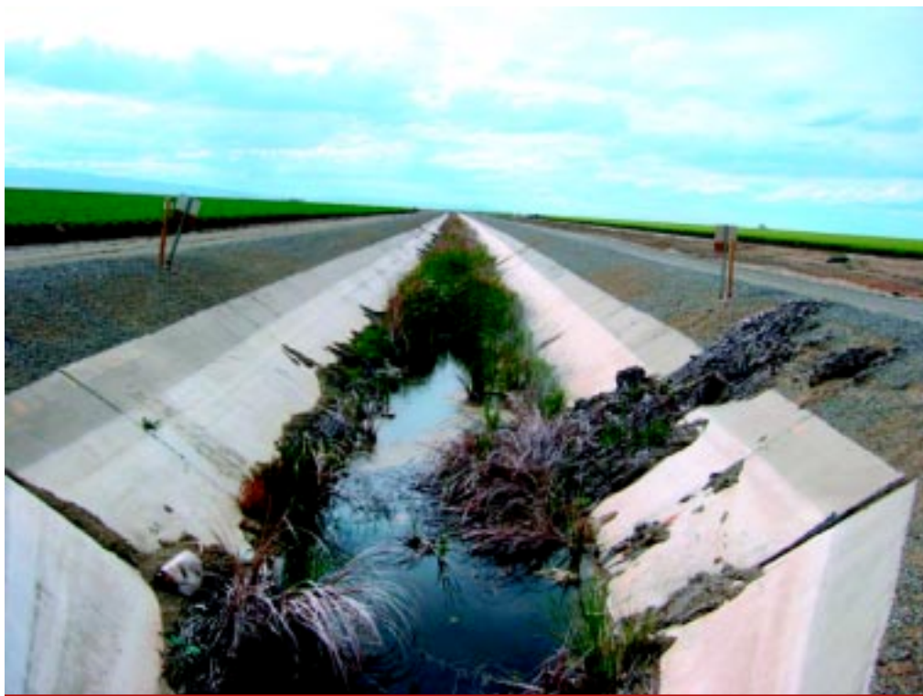
The San Luis Drain canal in western Fresno County, which carried selenium-laced drain water from the Westlands Water District to Kesterson in the early 1980s. Much of the canal was closed in 1986. A larger portion of the $80 million canal has not been maintained and has fallen into disrepair. The toxic salt buildup on the canal bottom was left in the canal and vegetation maintained by rainfall and seepage through the broken cement plates from adjacent irrigation has created a mini-habitat for wildlife which could be getting poisoned. Taxpayers foot the bill for this now unused linear toxic waste site. Photo by Lloyd Carter.
