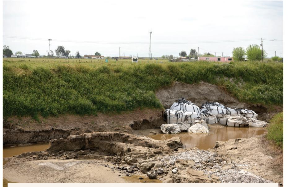
Huge sandbags were dropped by a Caltrans helicopter to keep this levee on the White River from being washed away by surging floodwaters.
