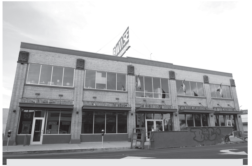
The Bitwise South Stadium Building a few weeks after the company imploded in 2023. Photo by Peter Maiden
