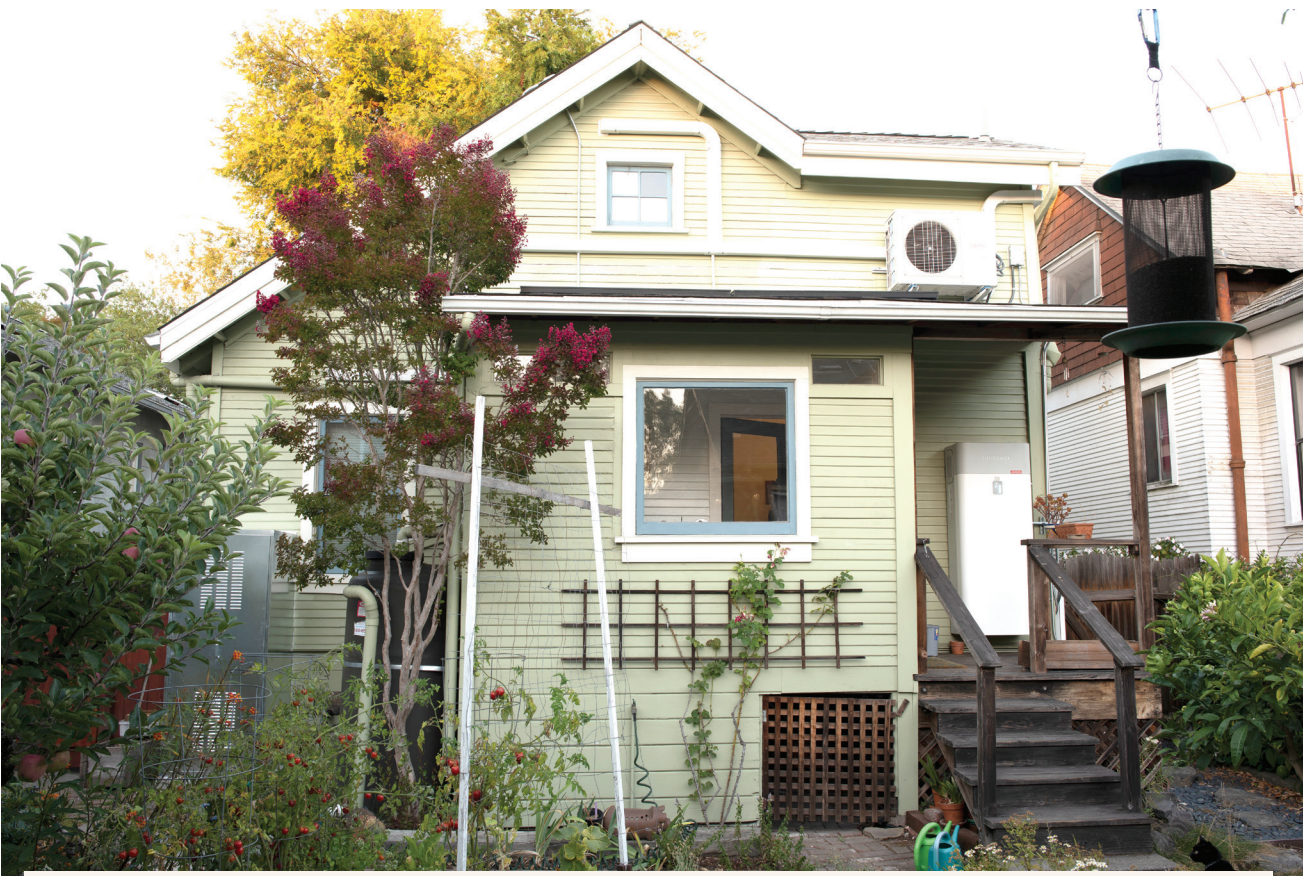
Shauna and Mark's green home. Attached to the wall on the second floor to the right is an HVAC unit, with conduits leading to three indoor heating/cooling units. On the porch is a battery for solar power, about the size of a small refrigerator. At the far left is a stainless steel cabinet inside of which is a water tank for the water heater. If you look carefully, next to the hot water tank, toward the porch, is a catchment tank for rainwater from the roof for watering the garden. Photo by Peter Maiden
