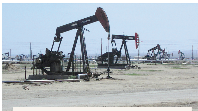
From Los Angeles to Kern County to the Bay Area, more than seven million Californians, totaling 18% of the population, live within a mile of at least one oil or gas well. Photo courtesy of The Commons
